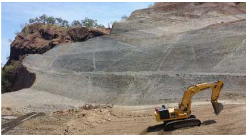
Image 2 – 80 tonne excavator in Stormwater Pond 3
