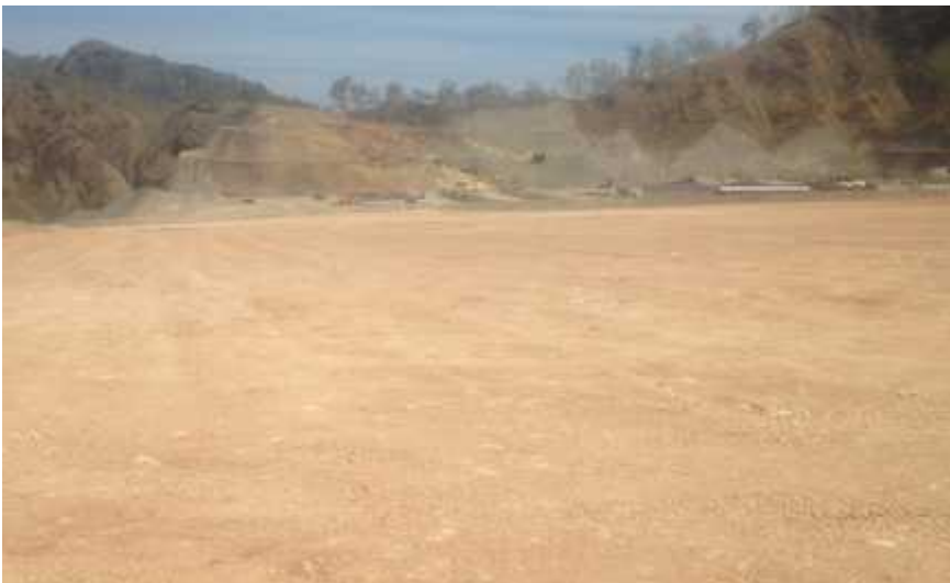
Image 4 – KKV Heap Leach Pad final level prior to lining – 25kt SX-EW site in the background
