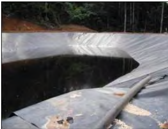
Figure 7. Completed new stormwater pond
