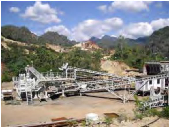
Figure 6. Refurbished crusher at Wetar
