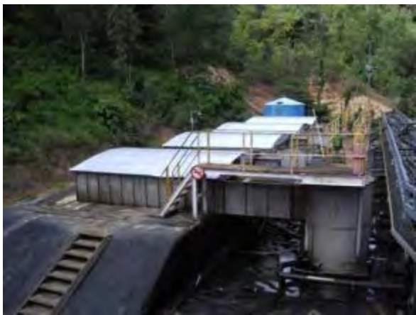
Figure 8. Covers on the SX plant
