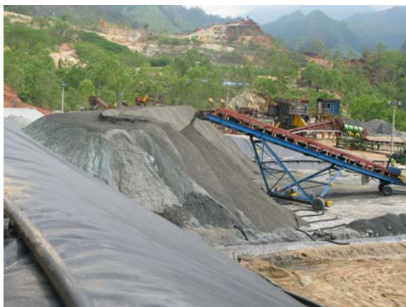
Ore stacking on demonstration heap, January 2009. Crusher in background. Photo: Finders.
