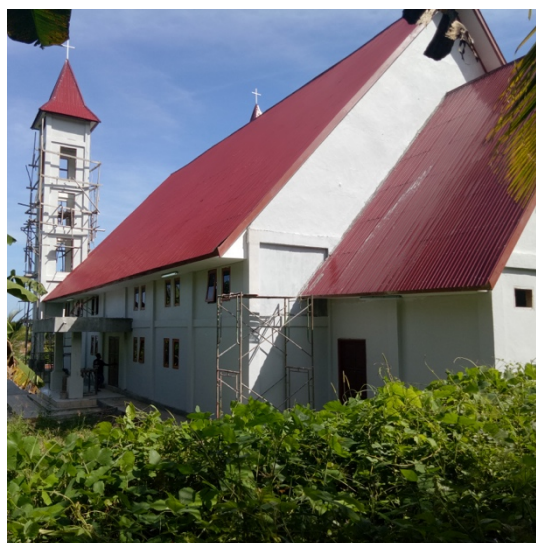
Image 5 –Uhak Church works nearing completion
