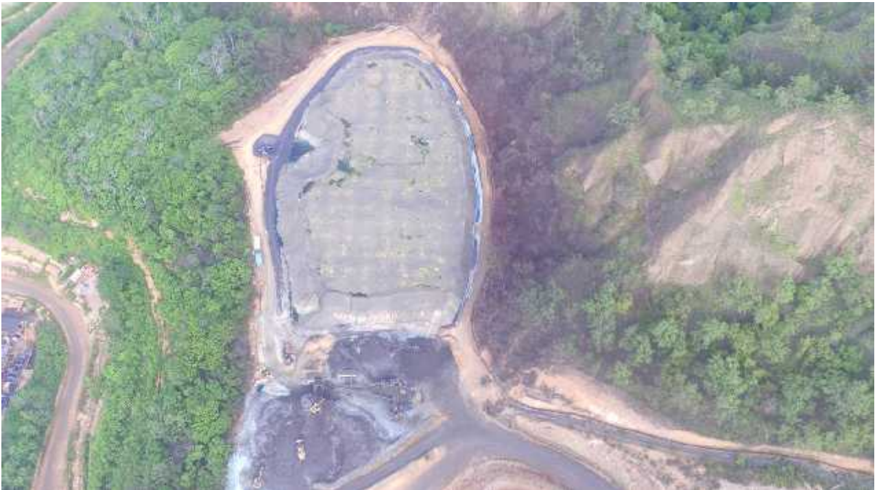
Image 3 – Crusher 21 and leach pad DP07
