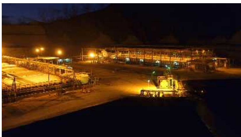
Image 4 –25,000 t.p.a. SX-EW plant at night
