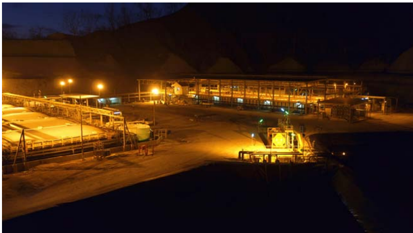
Image 4 – Aerial view of the 25,000 t.p.a. SX-EW plant at night
