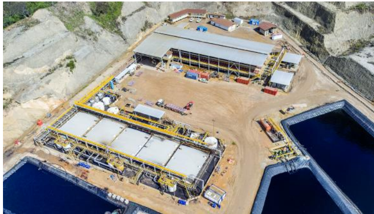
Image 4 – Aerial view of the 25kt SX-EW plant
