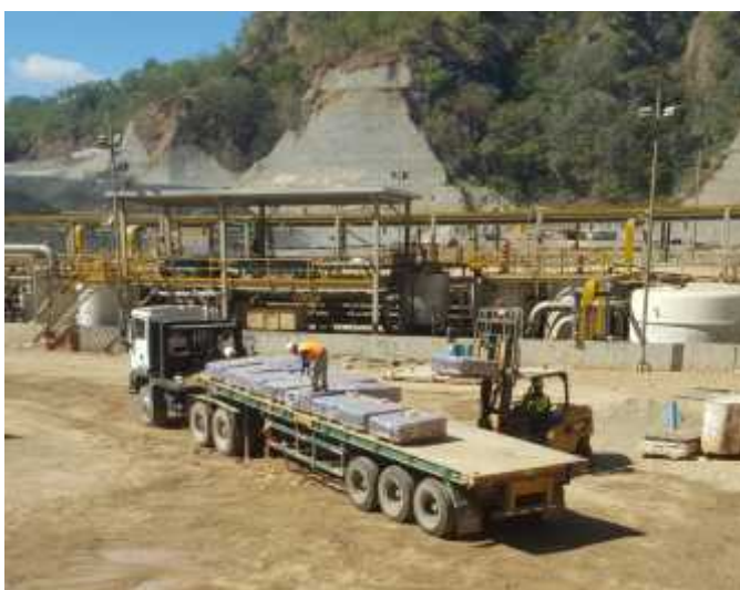
Figure 1: Pallets of LME Grade A copper cathode from the 25,000 t.p.a. SX-EW plant being loaded to truck.
