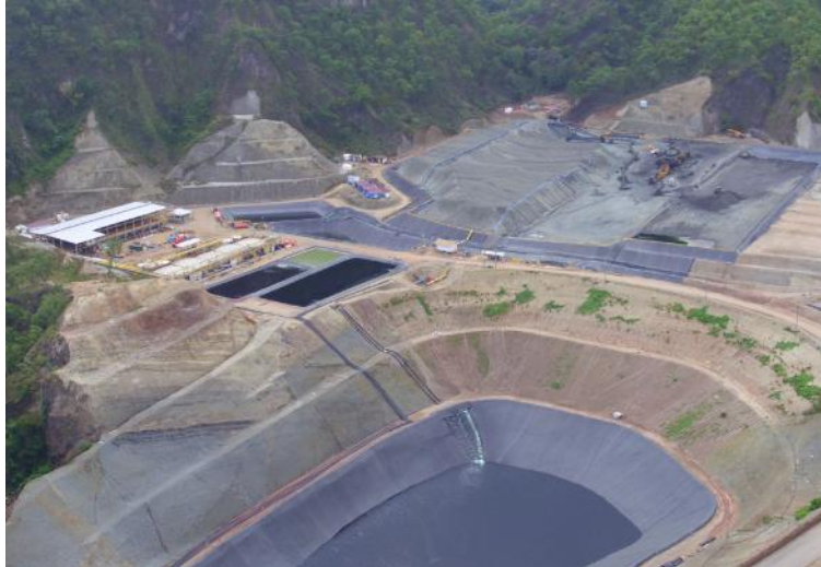
Image 4 - Aerial view of the 25,000 t.p.a. copper cathode SX-EW plant
