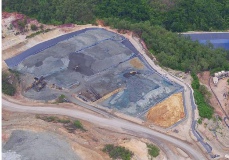
Image 2 – Aerial View of the Gold Pit Heap Leach Pad
