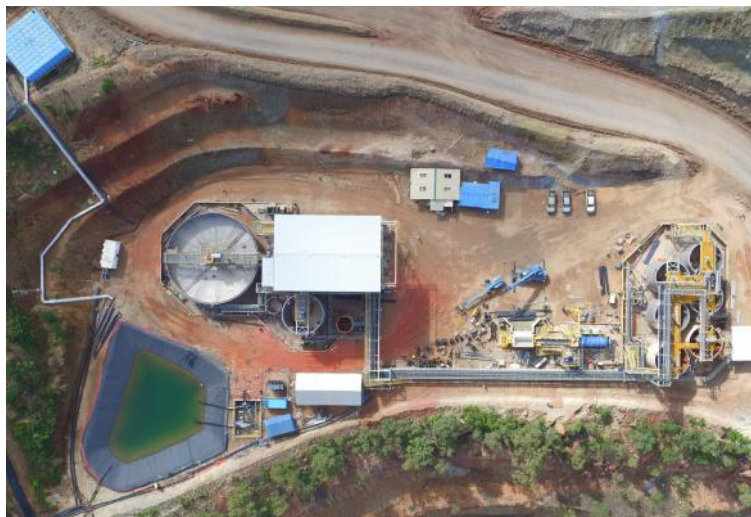
Image 5 – Aerial view of the Neutralisation plant
