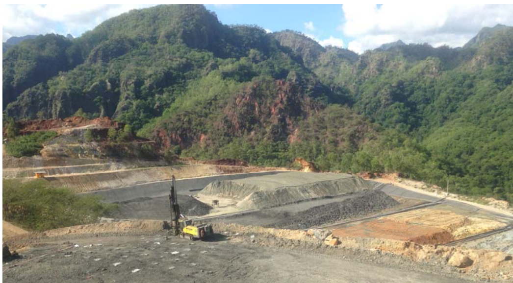
Image 1 – GPLP heap, broken ore stocks and limestone heap
