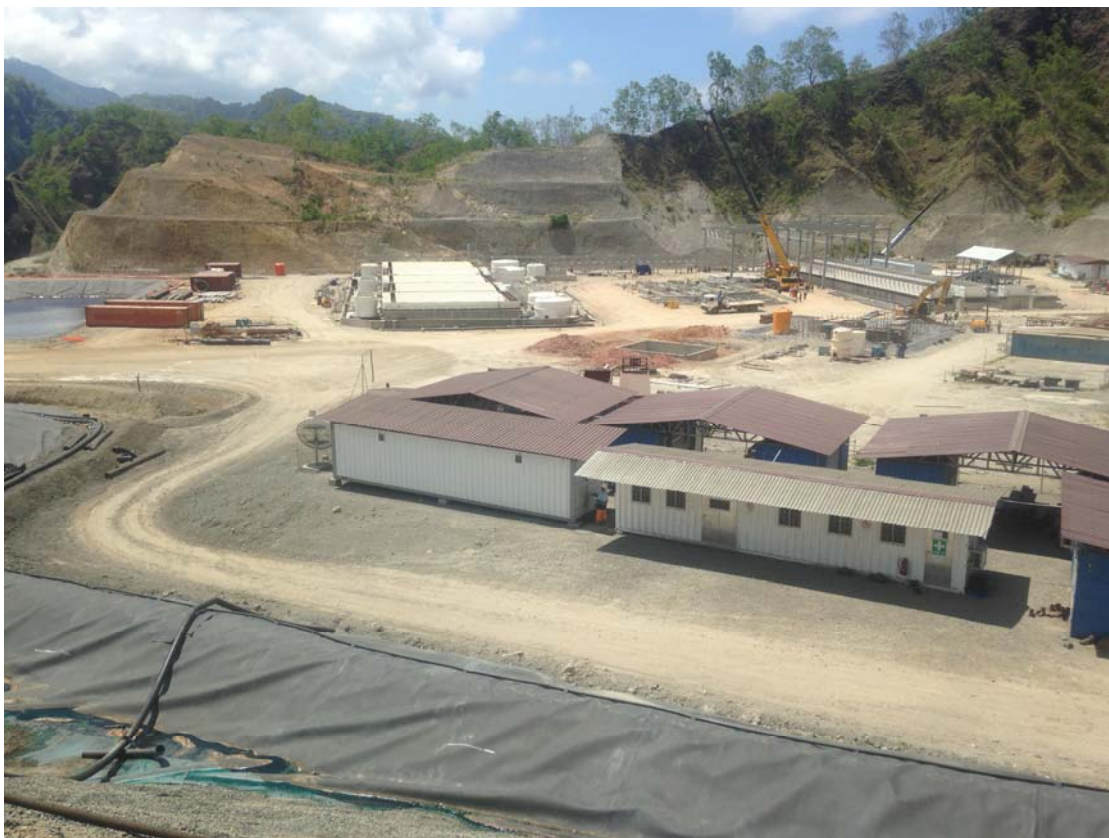
Image 4 – 25 kt plant construction from the KKV leach pad
