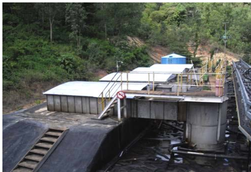
Figure 1: SX Plant at Wetar
