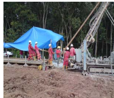
RC Drilling at Ojolali
