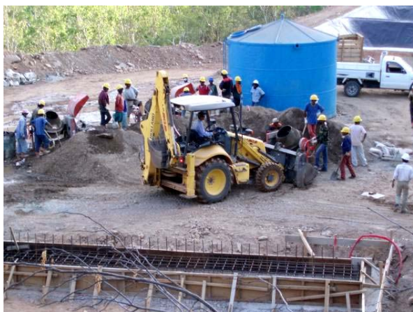
Last pour of concrete at SX location
