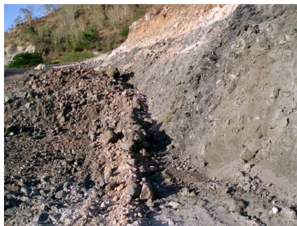
Pre-stripped test pit
