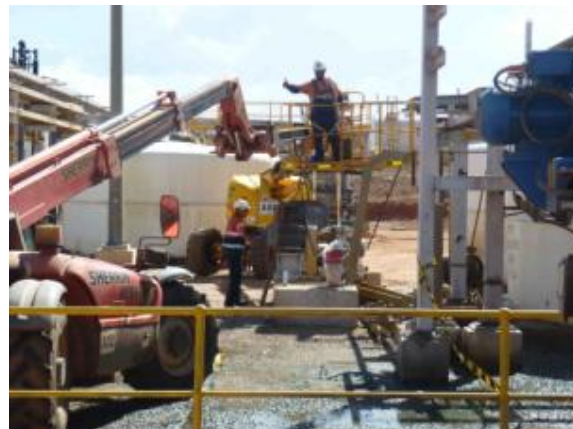
Fig 4: Equipment removal at Whim Creek
