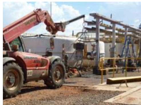
Removing pumps at Whim Creek
