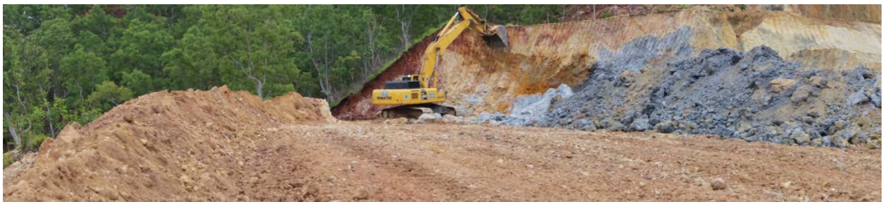
Photograph above shows the excavator at work on the KKV Access
