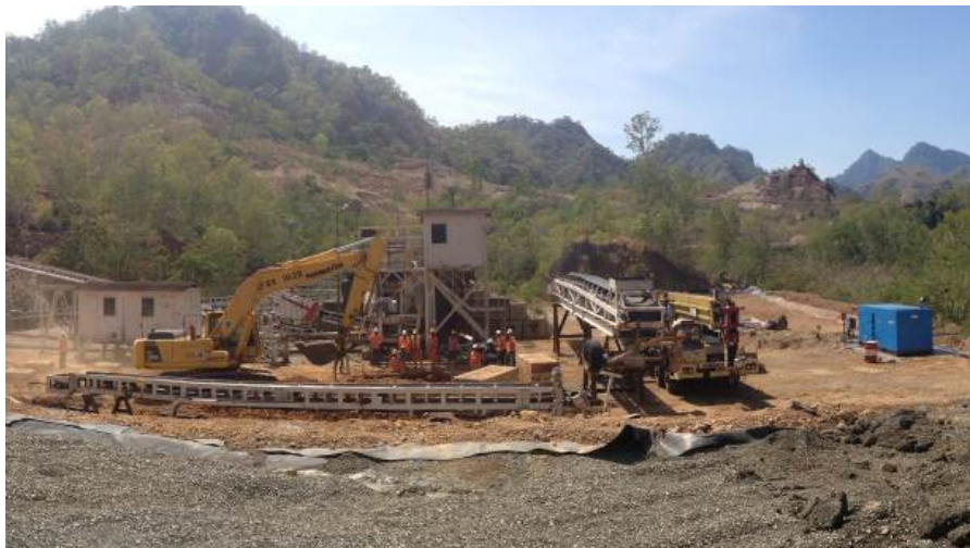
A construction team establishing the civil foundations for elements of the refurbished crushing circuit.
