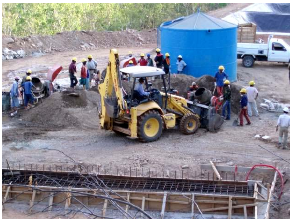
Last pour of concrete at SX location
