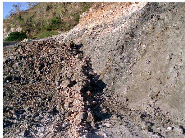
Pre-stripped test pit
