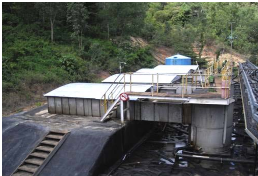
Figure 1: SX Plant at Wetar
