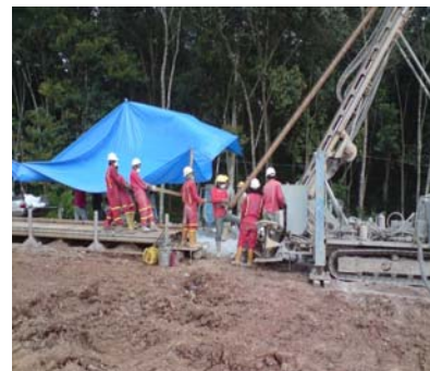
RC Drilling at Ojolali
